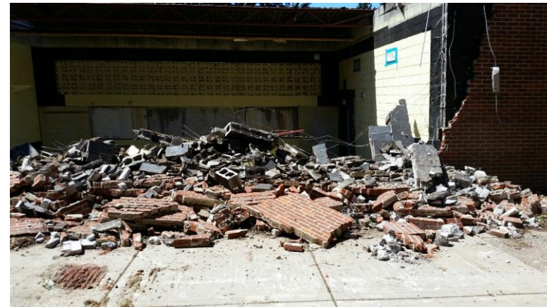
Phase I Music Room Demolition
