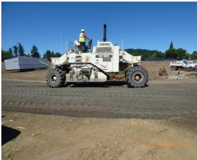
Asphalt grinding
