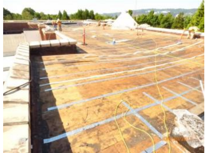
Buckman Roof/Seismic Work
