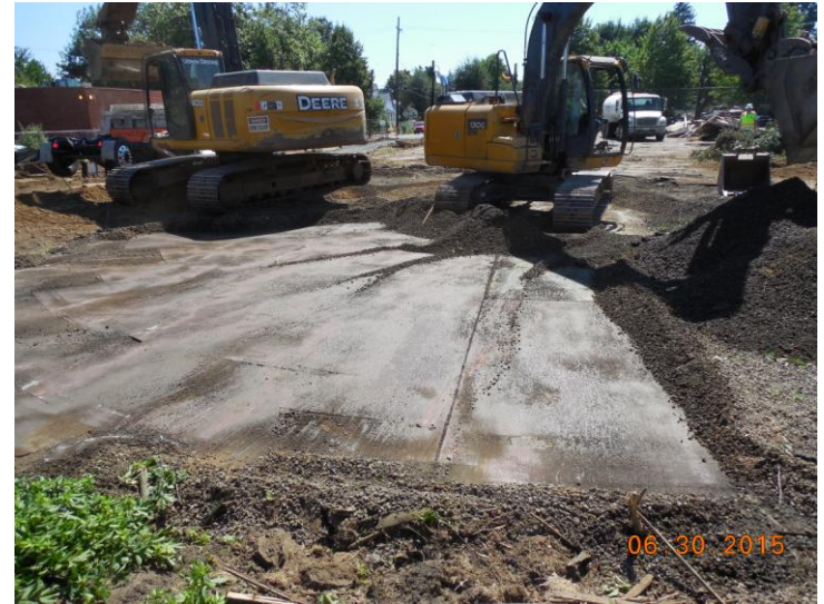
Concrete Under Tennis Courts
