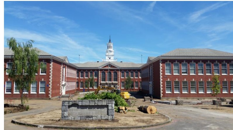
FHS Southern Entrance
