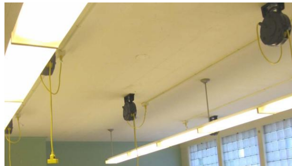
New Electrical Outlets at Peninsula
