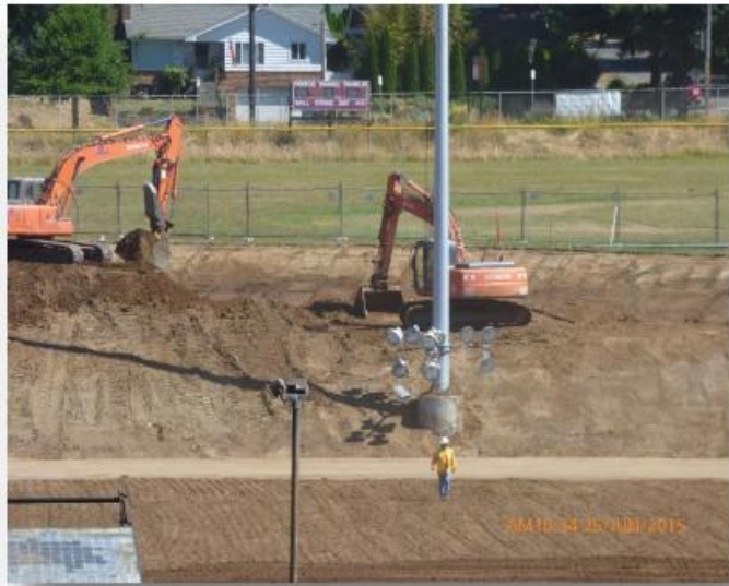
Cut and fill of earthwork on the field
